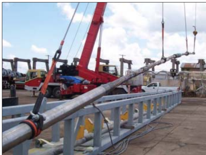
Onshore lift tests ensured the functionality of the compensating sling used for lifting the long bottomhole assembly offshore (Fig. 3).
